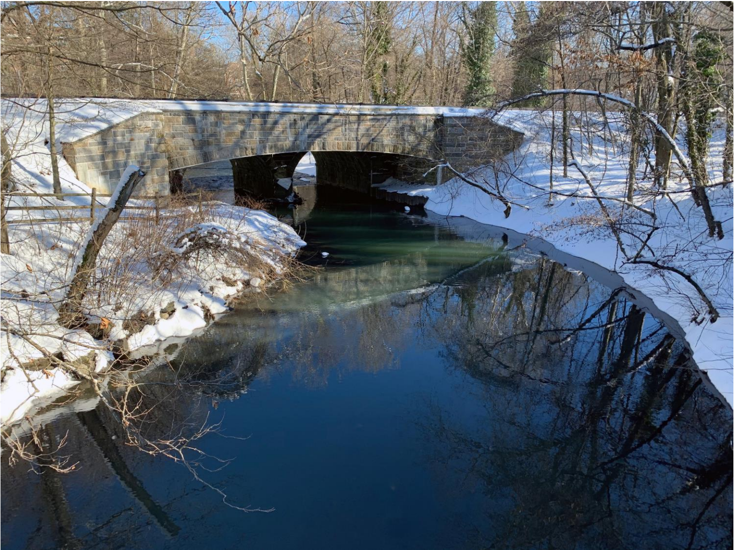
Midland Avenue Bridge over Bronx River
