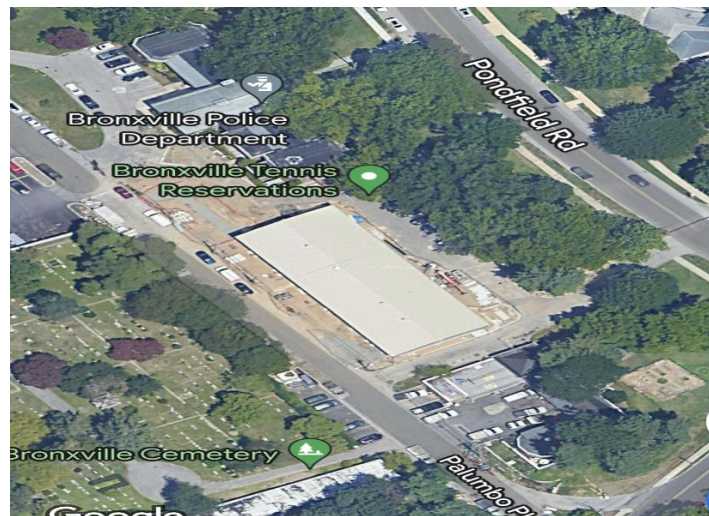
Roof of new Department of Public Works building
