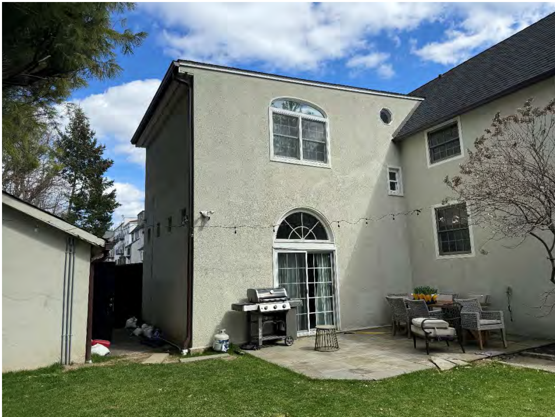
87 Kensington Rd (Rear View)
