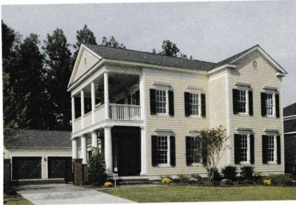
Montgomery, AL: Placed toward the rear of its lot, this garage at The Preserve does not detract from the appearance of the house it serves.
