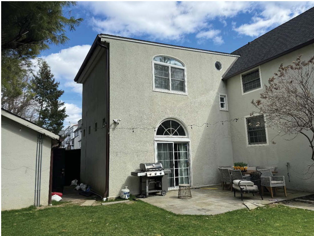
87 Kensington Rd (Rear View)
