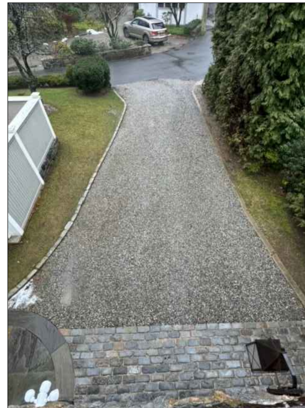
SITE PHOTO 4 – DRIVEWAY GARAGE VIEW 1
