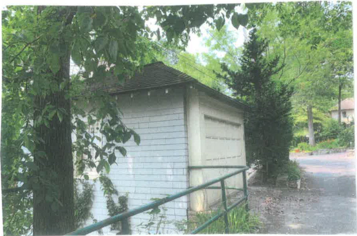
GARAGE OF 6 SUNSET ALONG STREET
