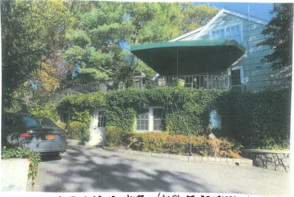
WEST SIDE OF HOUSE (AREA OF PROPOSED WORK)
