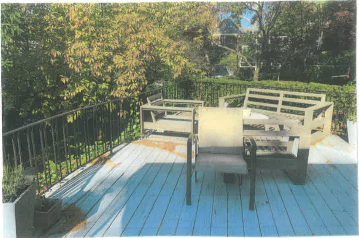
EXISTING DECK ABOVE REC. ROOM WITH POINTED EDGE
