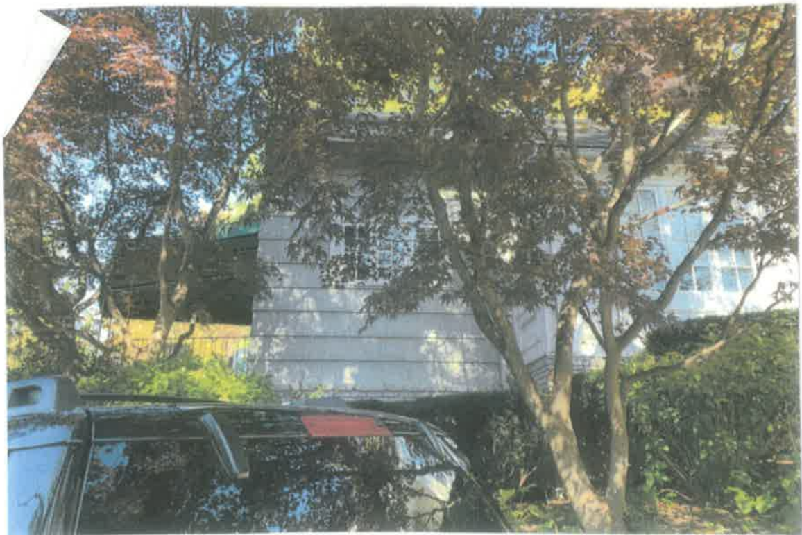
FRONT OF 21 SUNSET - WEST SIDE
