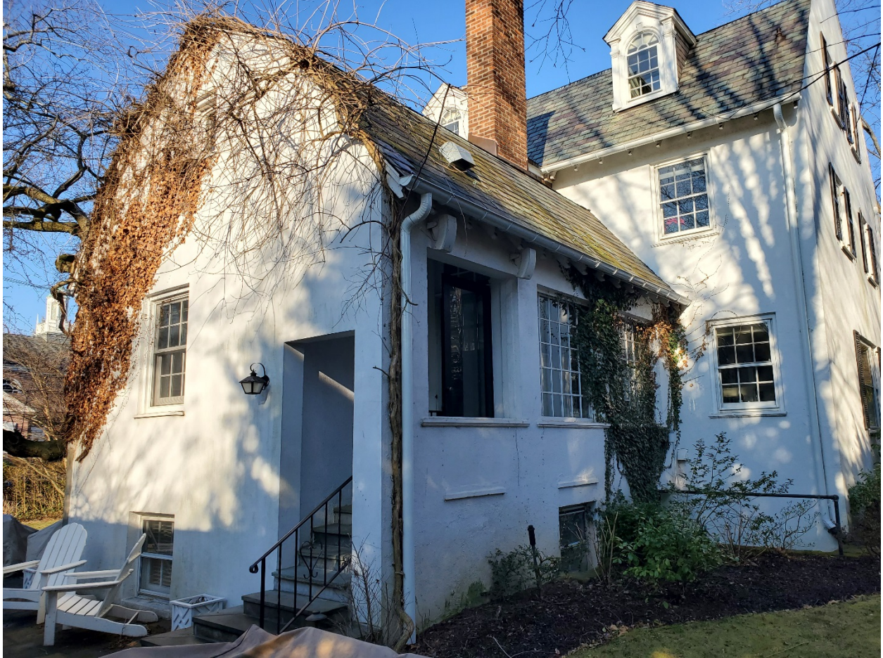
View of Southwest existing
