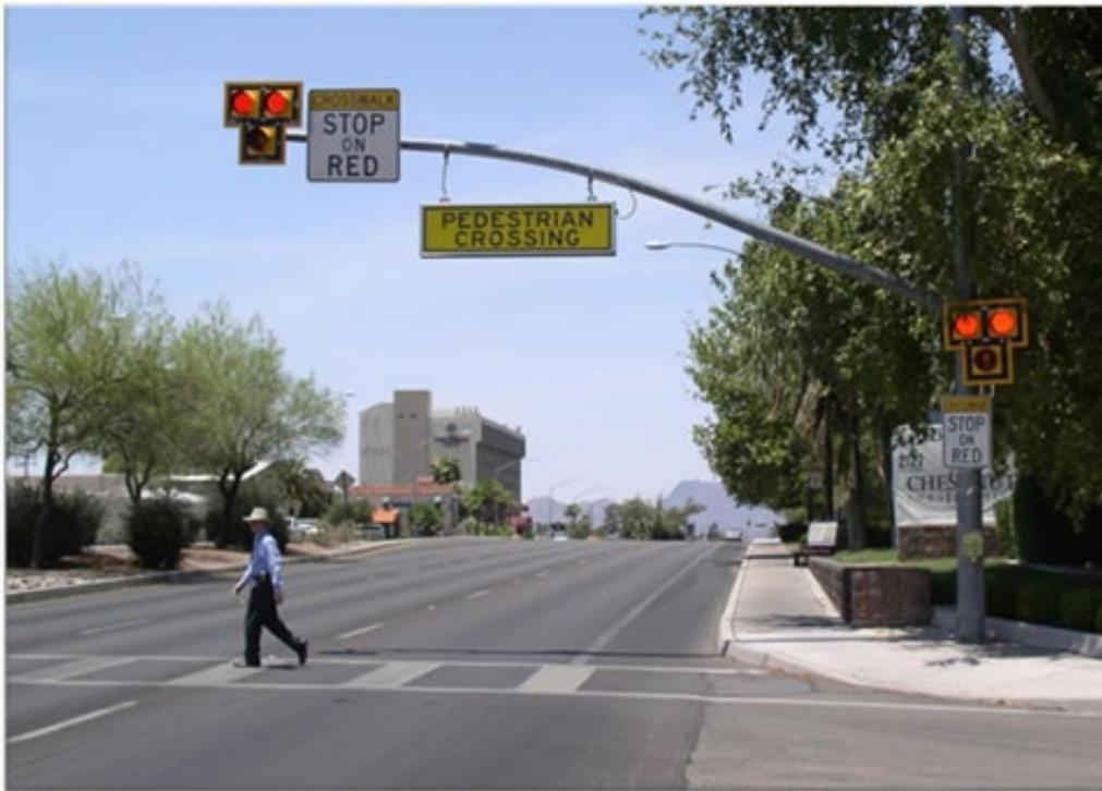
Figure 4F-1. Guidelines for the Installation of Pedestrian Hybrid Beacons on Low-Speed Roadways
